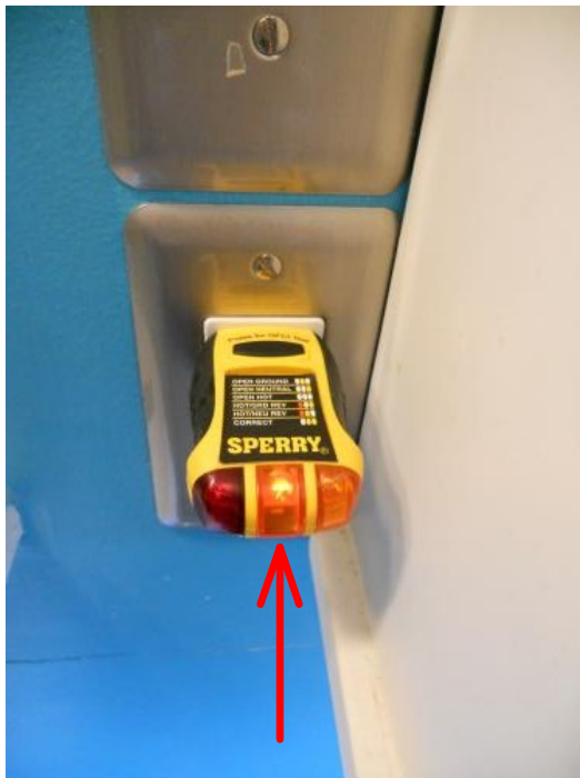
#19 Open or ungrounded connection.
